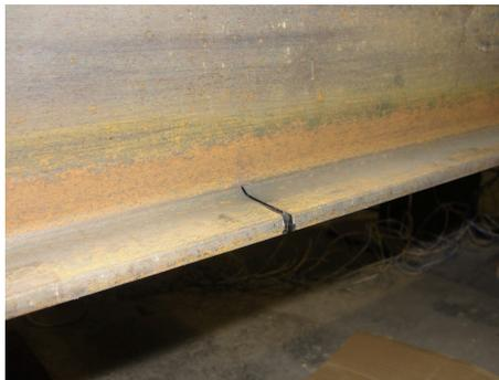
FIG. 7. Damage to the bottom flange.
