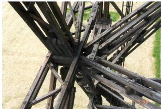
ensured continuity through the use of caps and inserts. Brass bolts and pins were used in all connections. The symbols R1, R2, ..., etc., and K1, K2, ..., etc. refer to the dimensions of particular elements of the tower (see Fig. 2).
