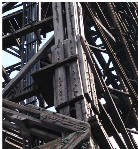
FIG. 6. A joint of the legs (photo: J. Broł 2002).
