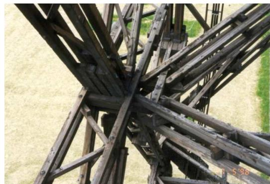
FIG. 8. Cross-sections of the four-bars diagonals [2].
