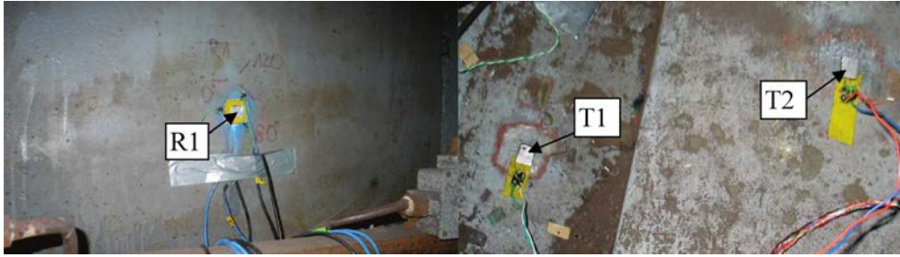
FIG. 12. Rosette R1 and single strain gauges T1 and T2 mounted crane structure.
