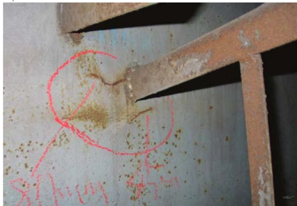
FIG. 4. Cracks weld of the crane beam stringer type "G" detected by the magnetic-powder method.
