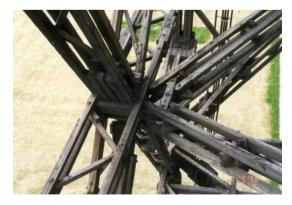
FIG. 9. View of the joint of diagonals, purlins and the spatial bracing (photo: A. Malczyk 1998) [2].
