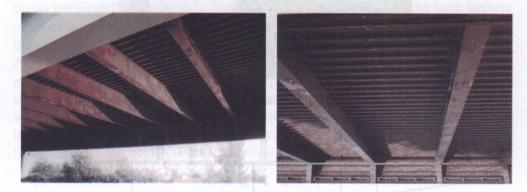
Fig. 4. Details of transverse cross-beams supporting the longitudinally stiffened plate and instrumentation.
