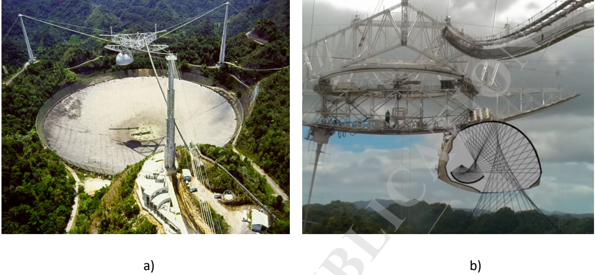
Fig. 19. (a) The spherical antenna of the radio telescope in Arecibo, Puerto Rico [20] (b) Reflectors of the Arecibo Gregorian Optics [21]
