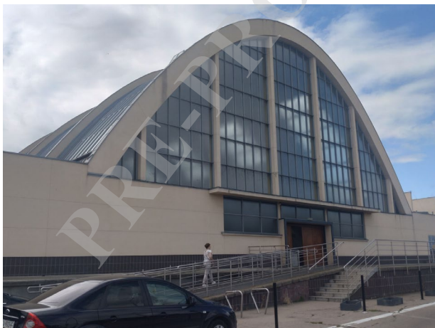
Fig. 16. The market hall in Gdynia with a parabolic roof, built in 1938 in the constructivist style. Photo by A. Kulowski
